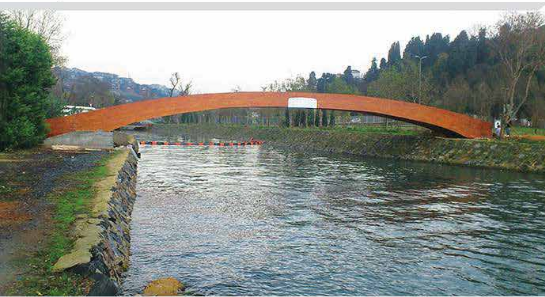
TBMM KÜÇÜKSU KASRI - KÖPRÜ 36 METRE
